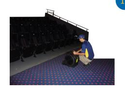
Dry the armchairs for at least 3 hours with the air turbine, changing it from place to place all over the auditorium to accelerate the process.
