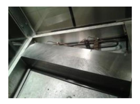
Step 10- Once secured the protector, the refractory top is placed again, the resistance is turned on and we wait for it to warm again.
